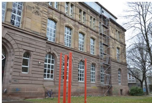
Figure 1: The north-east (NO) façade of HFT
