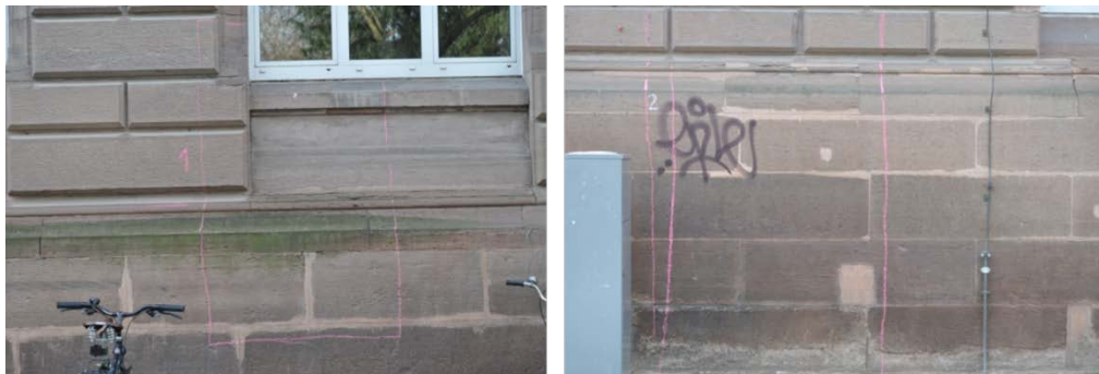
Figure 2: Two areas on the façade (left: area 1, right: area 2)
