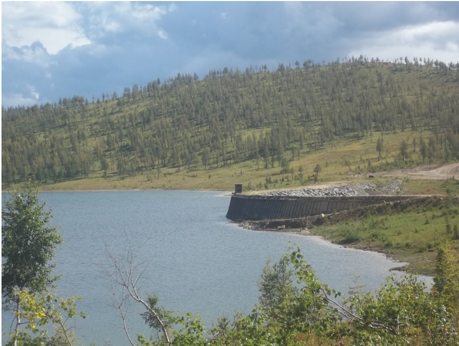
Figure 1: the Malo-Ulbinsky reservoir rock-fill dam
