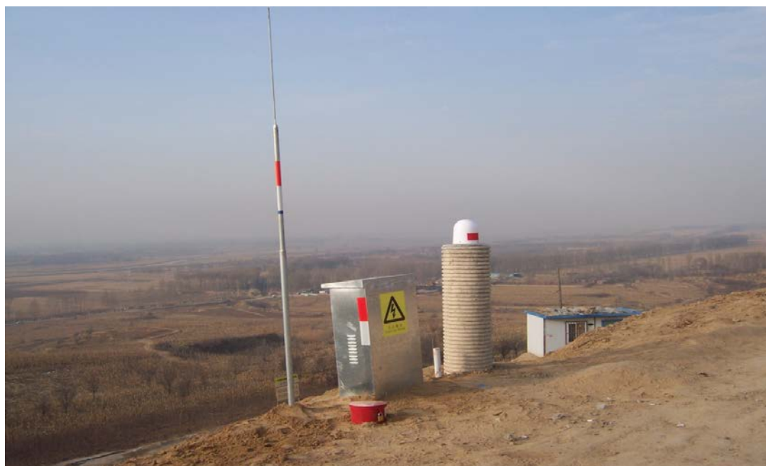
Figure 8: A typical switching antenna monitoring point with data collection cabinet and osmometer (red cylinder is the cover of osmometer pipe)
