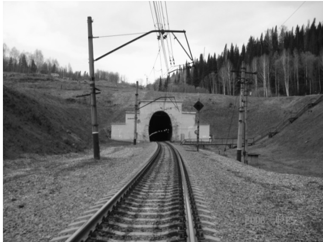
Figure 1: A portal of railway tunnel in Kemerovo Region
