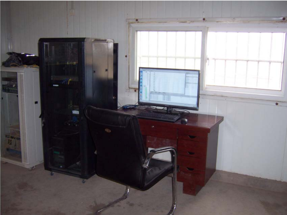
Figure 10: Central monitoring room
