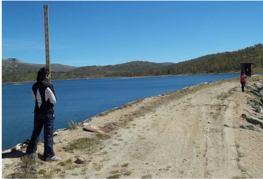
Figure 5: Marks levelling at the dam crest
