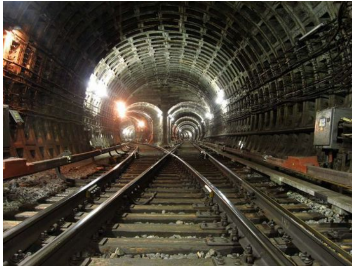
Figure 2: A view of the Novosibirsk subway tunnel.
