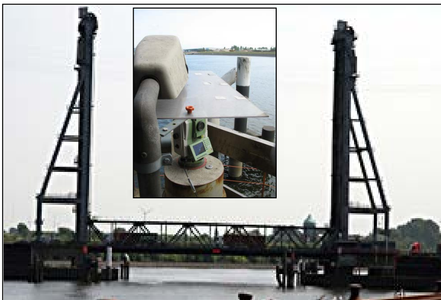
Figure 8: GOCA project Rethe lift-bridge maintained by Hamburg Port Authority (HPA) in the Hamburg port. Building monitoring during the construction of a new bridge close aside. Middle: installation of the total station (TPS) sensor.
