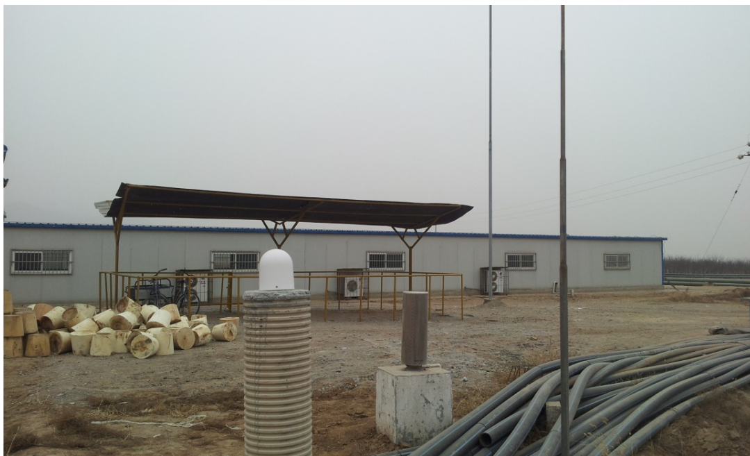
Figure 7: Base point and the central monitoring room behind
