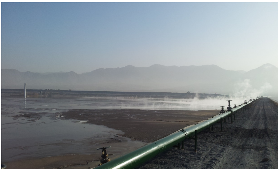
Figure 6: A view of this 2000 meter reservoir dam
