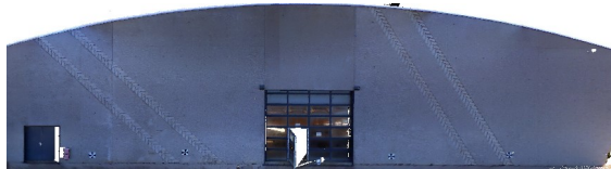
Figure 7: Scanned wall from Trimble X7.
