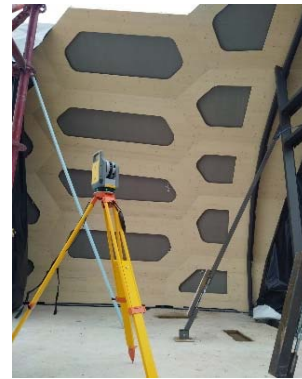
Figure 5: TLS measurements of timber shell
